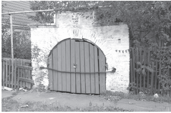
Gated entrance at street level to stairs leading down to an underground warehouse.
