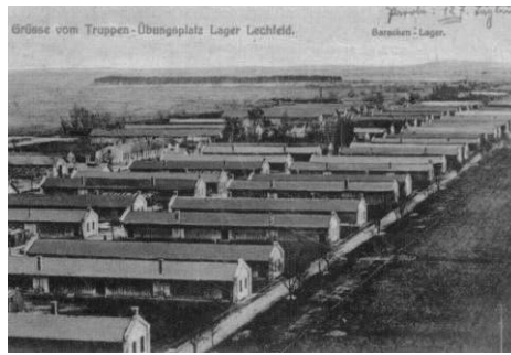
Army barracks in Lechfeld
