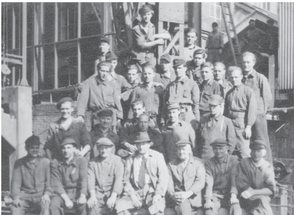
Photo 5: Men of the Gronau camp were put to work repairing war-damaged buildings, like the M. van Delden Factory pictured here. Photo credit: Peter Kroeker photo collection.
